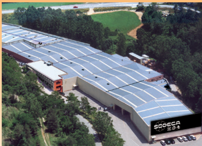
SODECA S.L.U. main facilities in E-08580 SANT QUIRZE DE BESORA
